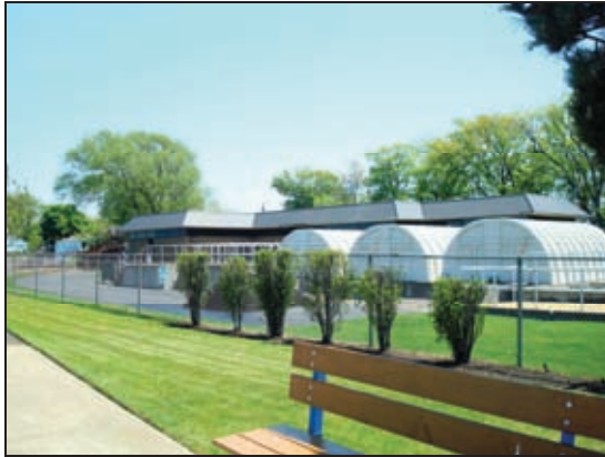
Village Sewage Treatment Plant
