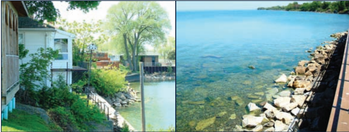
Shoreline Erosion Protection
